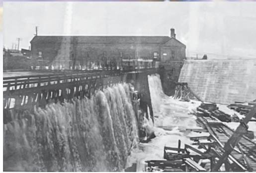
Construction area for stone dam showing new retaining wall from canal gatehouse to new dam. c1892-1900
