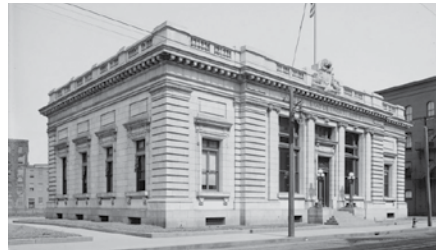
The former post office on Main Street, between Dwight and Race Streets in Holyoke, circa 1908.
